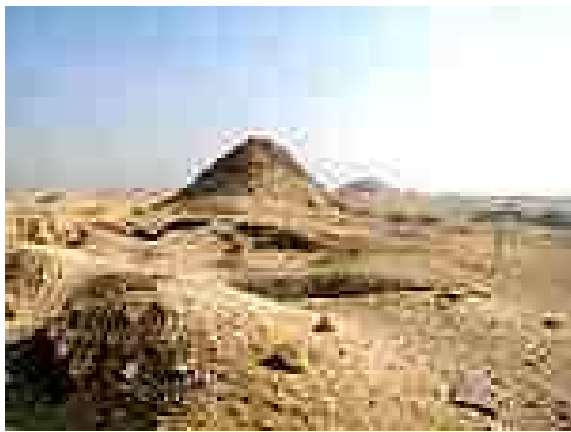
Userkaf's pyramid: Base: 73.3 meters Height: 49 meters Angle of inclination: 53 degrees Saqqara
