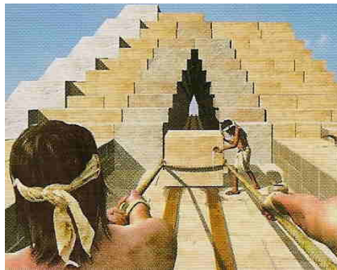
The blocks weighing several tonnes were pulled up via the interior ramp.
