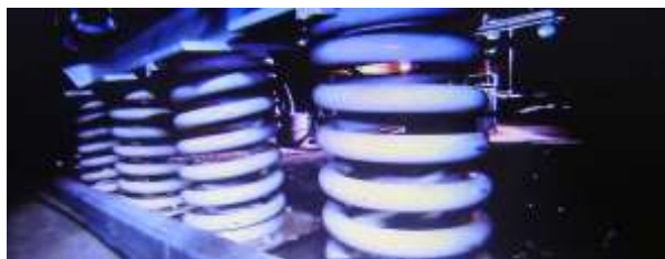
The Cheyenne bunker has more than 1,300 springs like these below the buildings.
